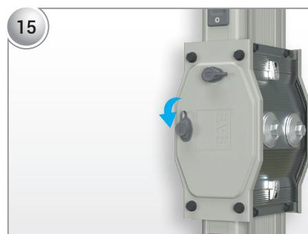
Once the injection process is complete, close the plastic cover and finalize the installation.
